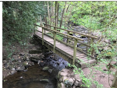
Bridge across Gill Beck
