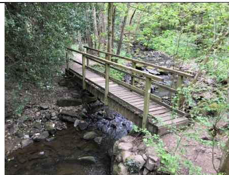
Bridge across Ghyll Beck
